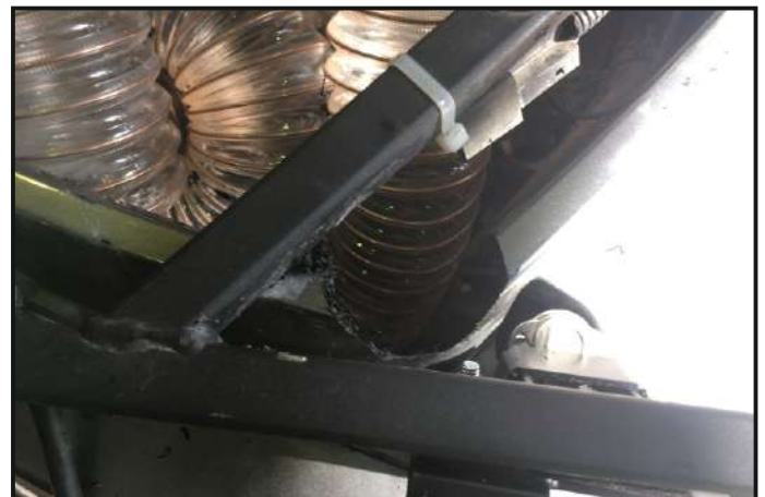
Drill a hole in the plastic panel d55-60mm
